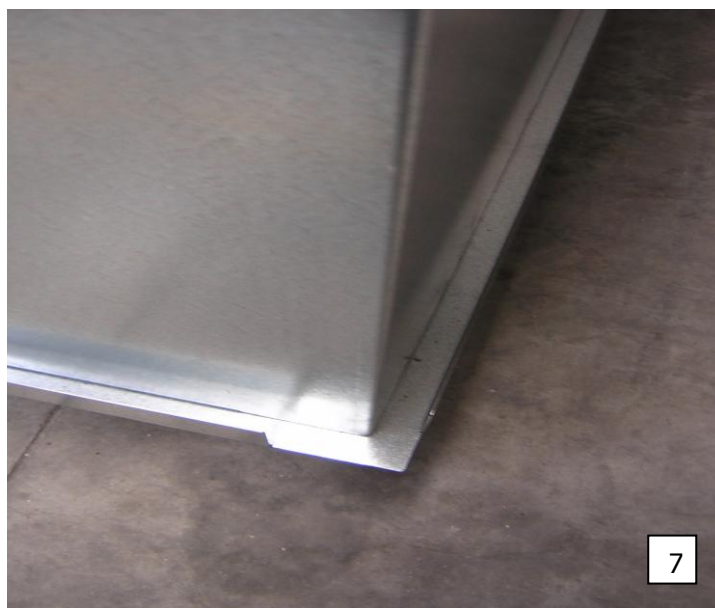
Profiled section for fixing of insulation
